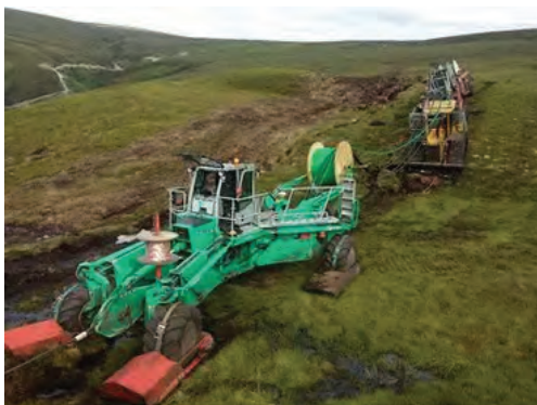
Laying system in mud and bog areas
