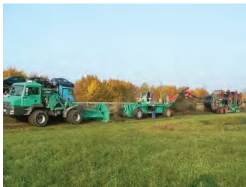
Laying of power cable
