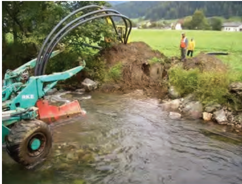
Laying pipes through watercourses
