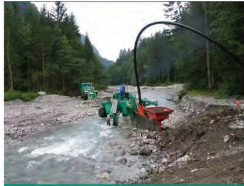
Laying system on rocky ground
