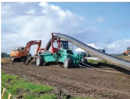
Laying of gas- and waterpipes
